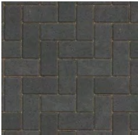
Charcoal block paving to parking bays
