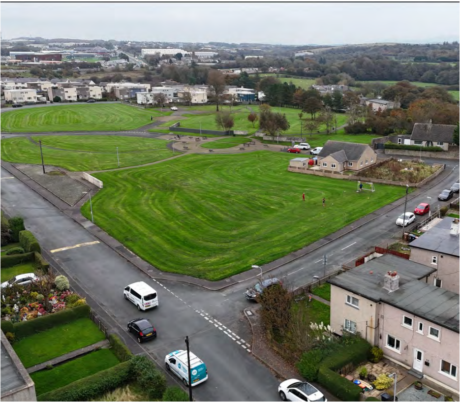
Arial View of Site From South West
