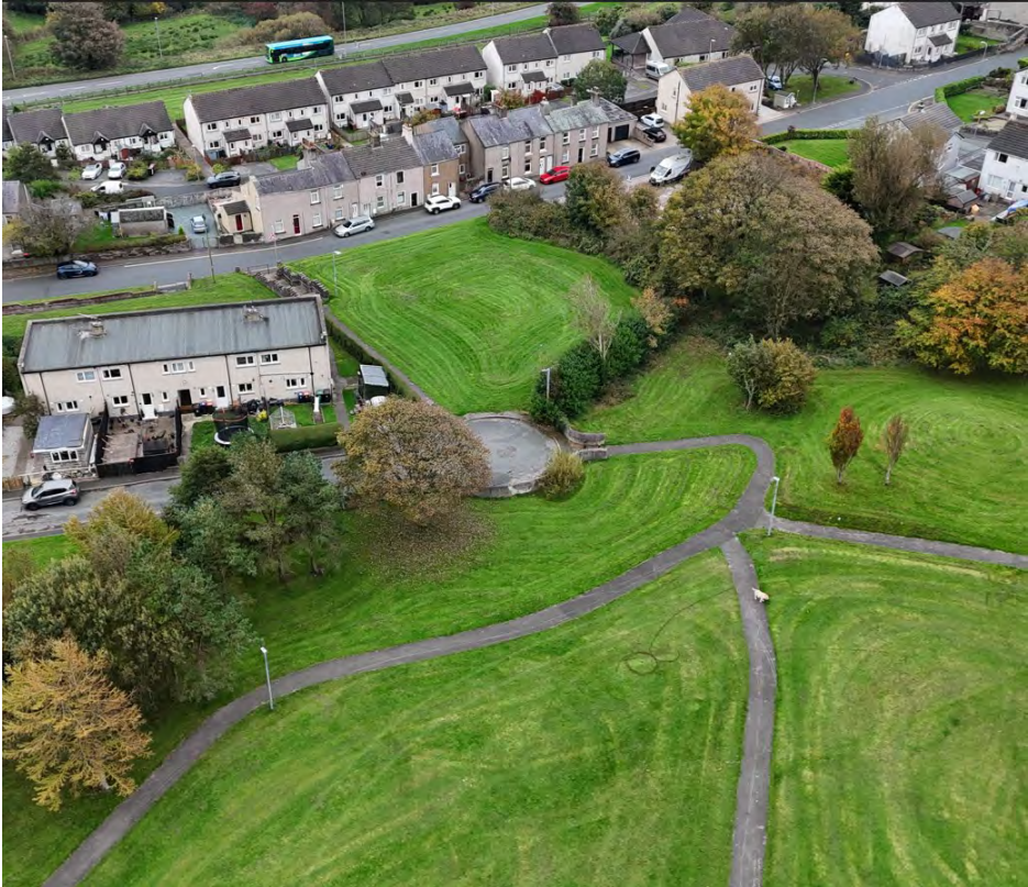
Arial View from North West
